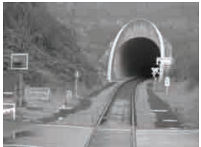
Büdesheimer Tunnel (Foto: Hollowpoint)
